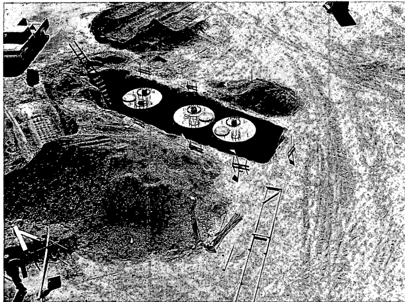
Fig. 2—Cells before backfilling and placing valves.
